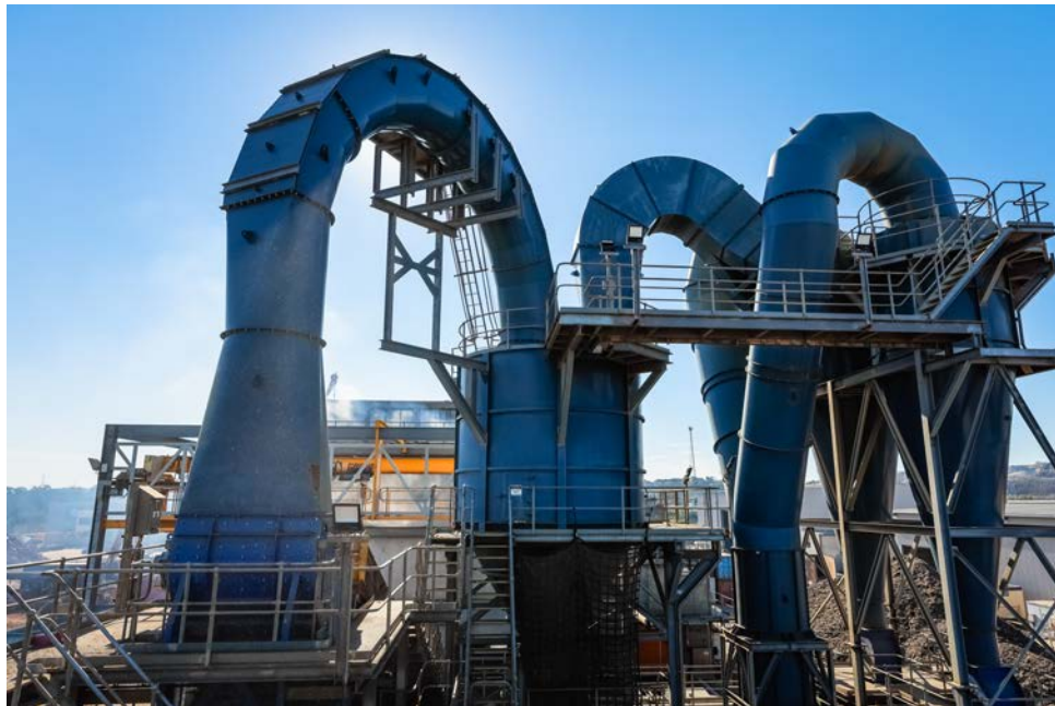
Sims Metal Kwinana, Western Australia
