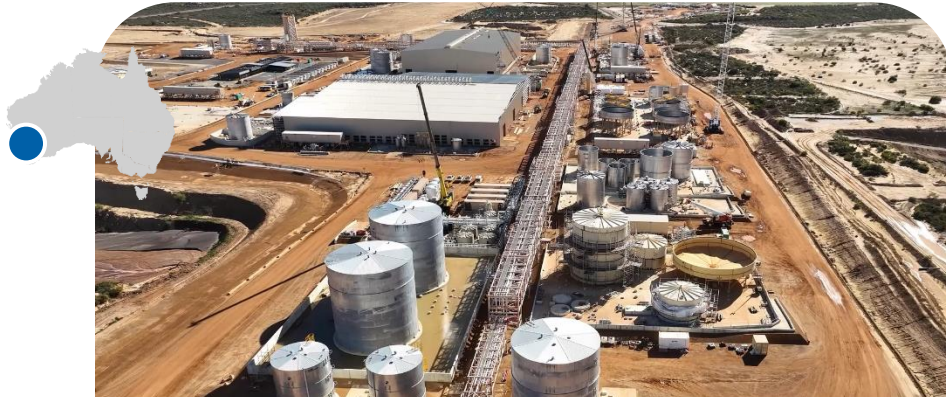
Eneabba rare earths refinery
