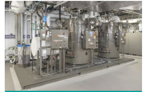
Vertical Steam Boiler
