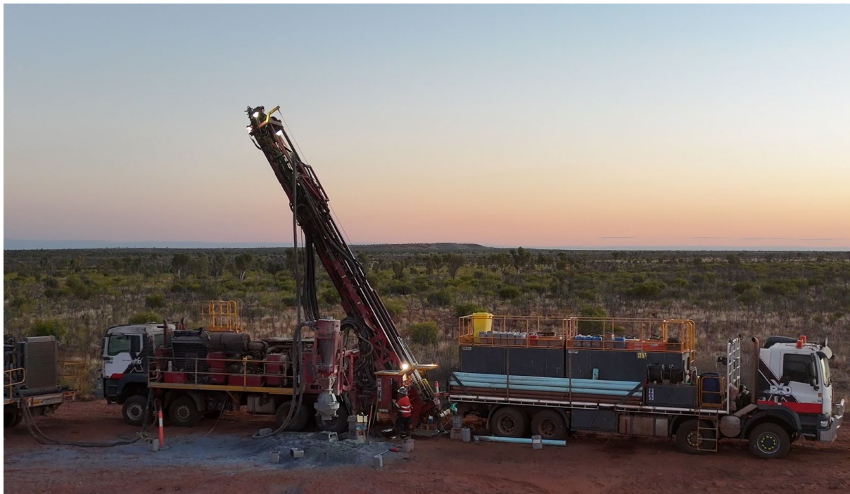
Figure 5. Drilling on-going at the Coogan Cu-Au Prospect, targeting recently identified IP chargeability anomalism.
