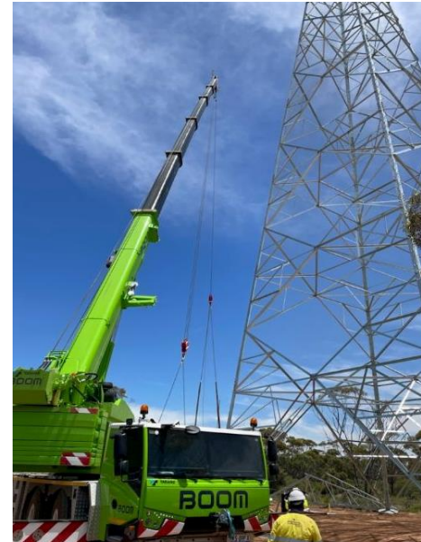
Hume Link West Transmission infrastructure 120t–250t cranes
