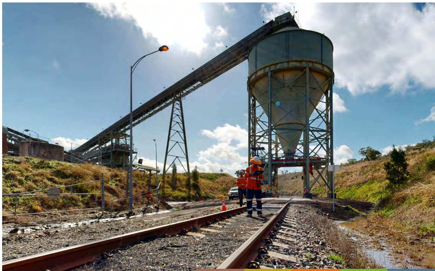
Track inspection, New South Wales
