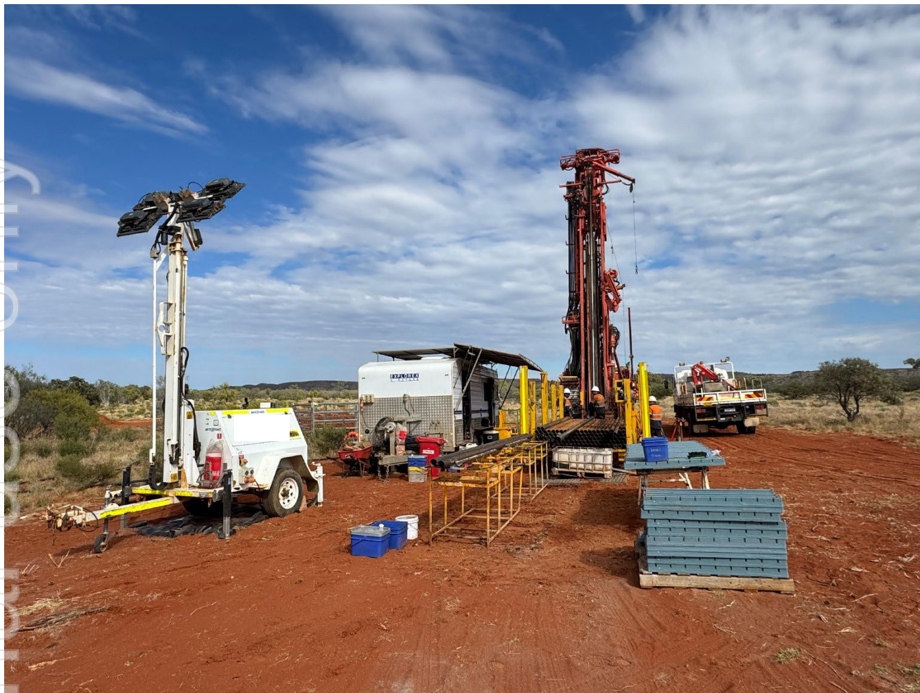
Figure 2: Drilling at Jervois Site
