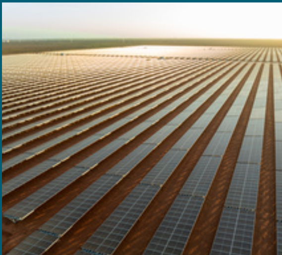
Image: Port Hedland Solar Farm, WA
