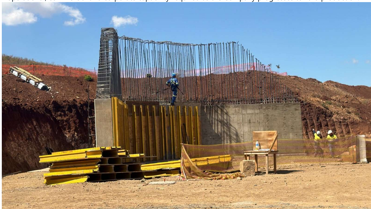
Picture 9. ROM pad civils advancing
