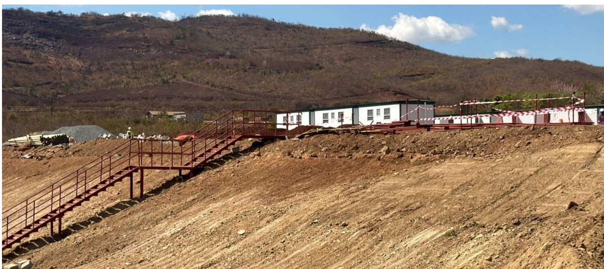
Picture 6. Phase 2 accommodation camp extension
