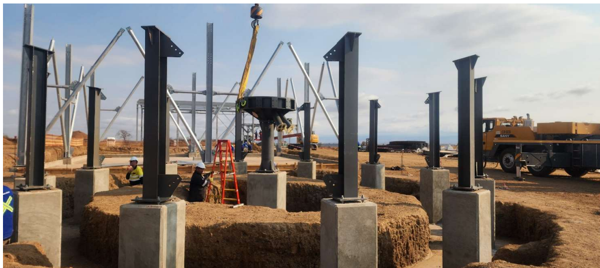
Picture 3. Thickener civils and structural installations
