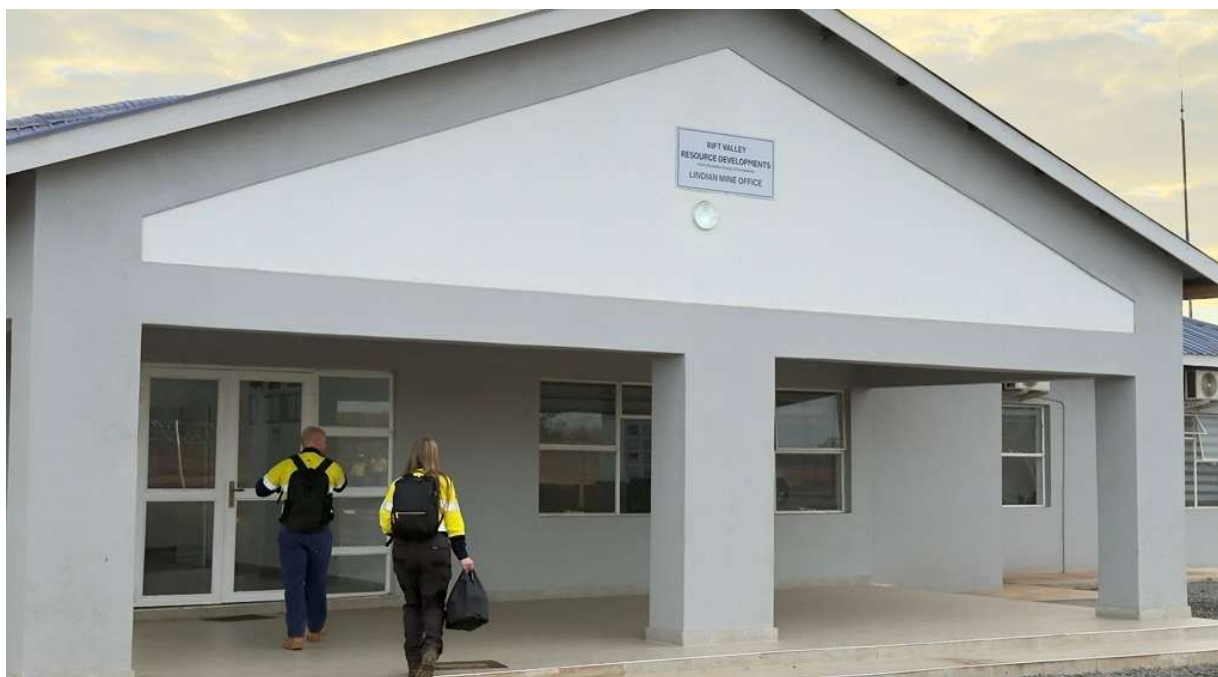
Picture 1. Kangankunde Mine Office
