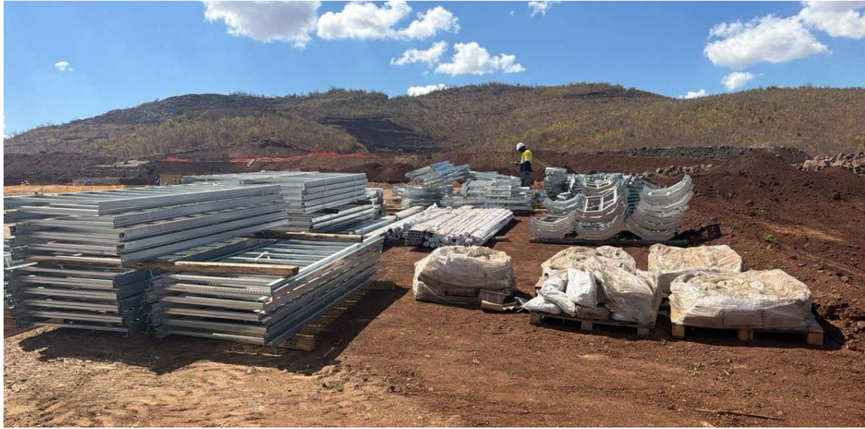
Picture 12. Plant cable recking delivered
