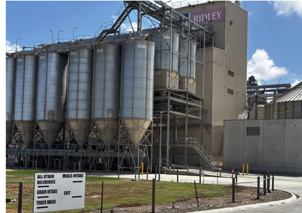
Lara Feedmill debottlenecking: new press installed to deliver 50kT annual additional capacity
