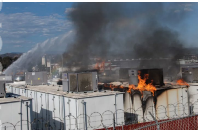
Escondido, California (September 2024): A BESS fire at a substation resulted in significant damage. The incident involved overheating of battery cells. Source: https://eticaag.com/thermal-runaway-in-battery-energy-storage-systems-bess/
