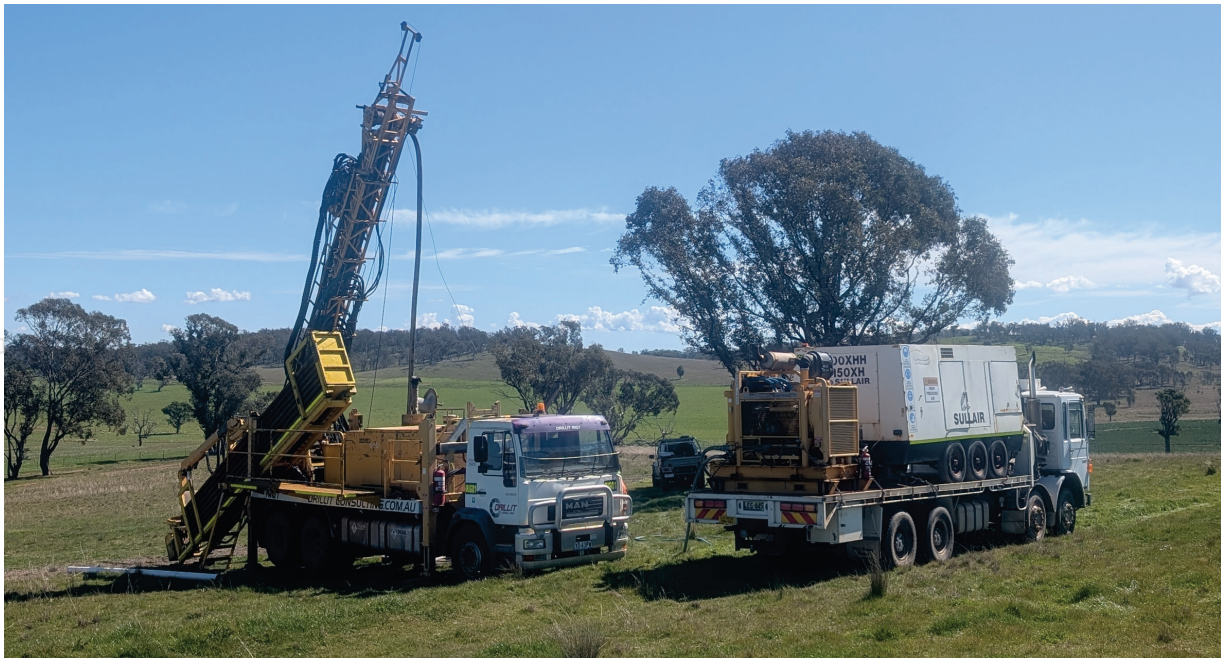
Photo 1. Drilling commenced at Dunedoo Project
