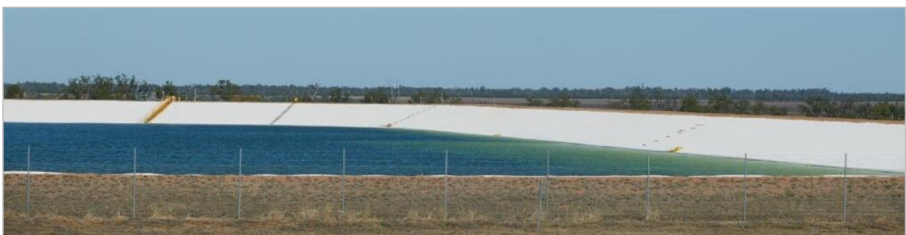
Figure 3.1 CSG brine dam (GISERA, 2026)
