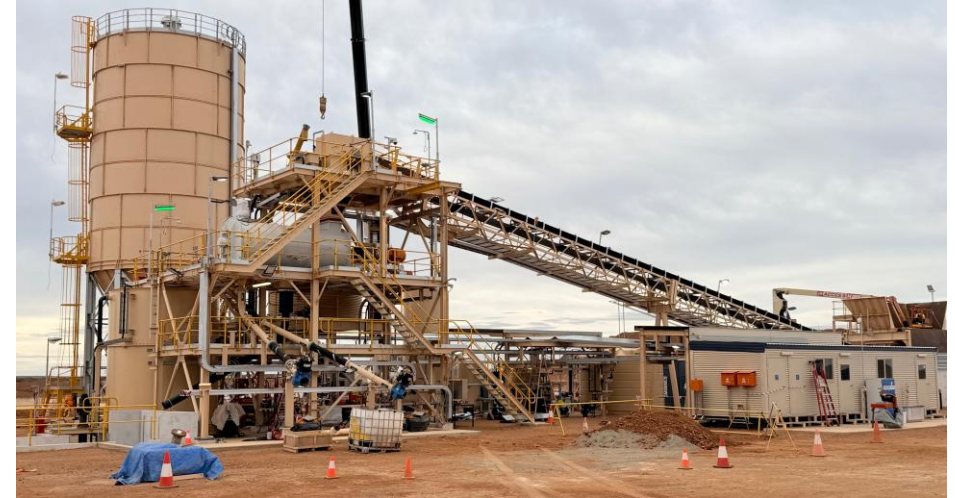
Paste plant nearing commissioning
