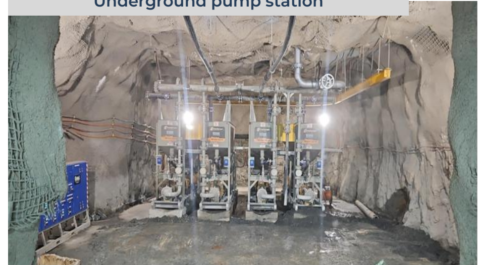
Underground pump station
