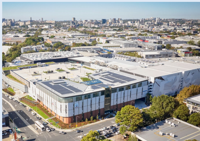
Ascent Logistics Centre, Alexandria (CLP)
