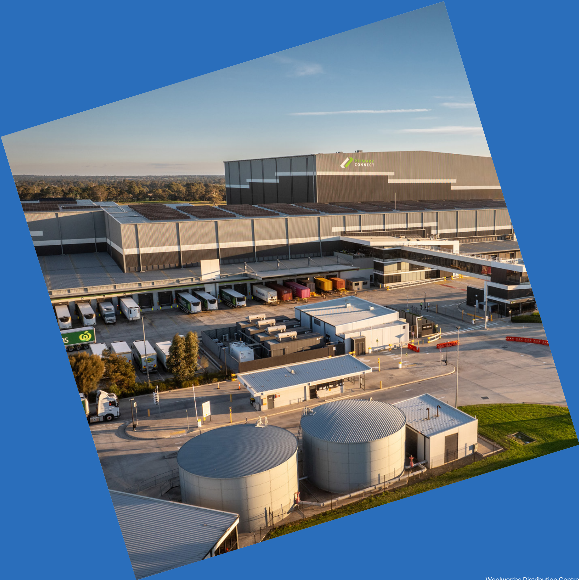
Woolworths Distribution Centre Melbourne, VIC Wurundjeri and Bunurong land
