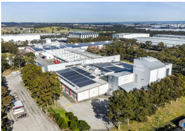
Solar panels on Huntingwood Distribution Facility NSW Darug land
