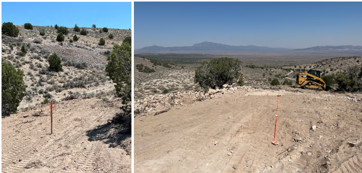
Figure 2- Drill pad preparations- North Star Prospect
