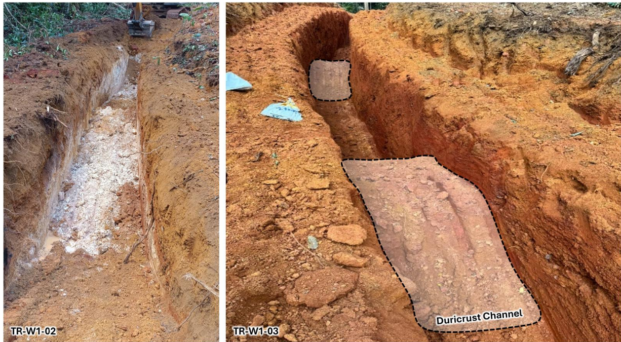
Figure 6: Shallow trenches TR-W1-02 (left) and TR-W1-03 (right) in upper lateritic profiles.
