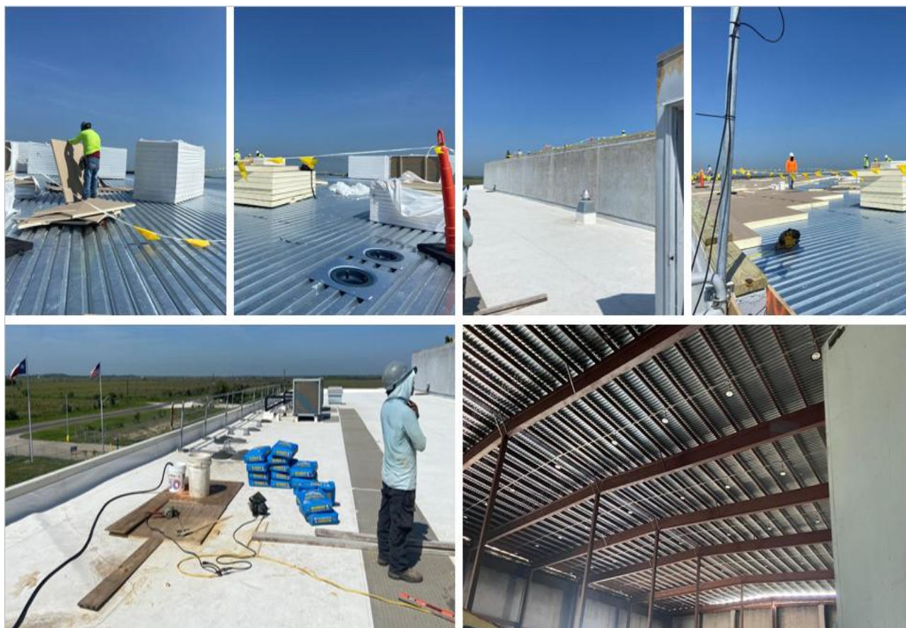
Figure 3: Area 140 Roof – August 2026
