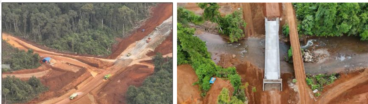
Sampala Mine construction activities
