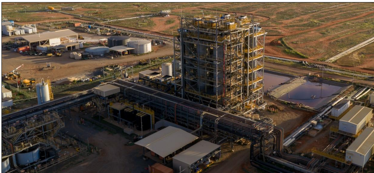
Figure 27: Photo of existing Honeymoon processing plant
