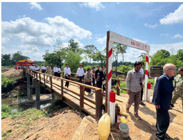
Figure 46 | The new bridge at O’Pungtou River crossing
