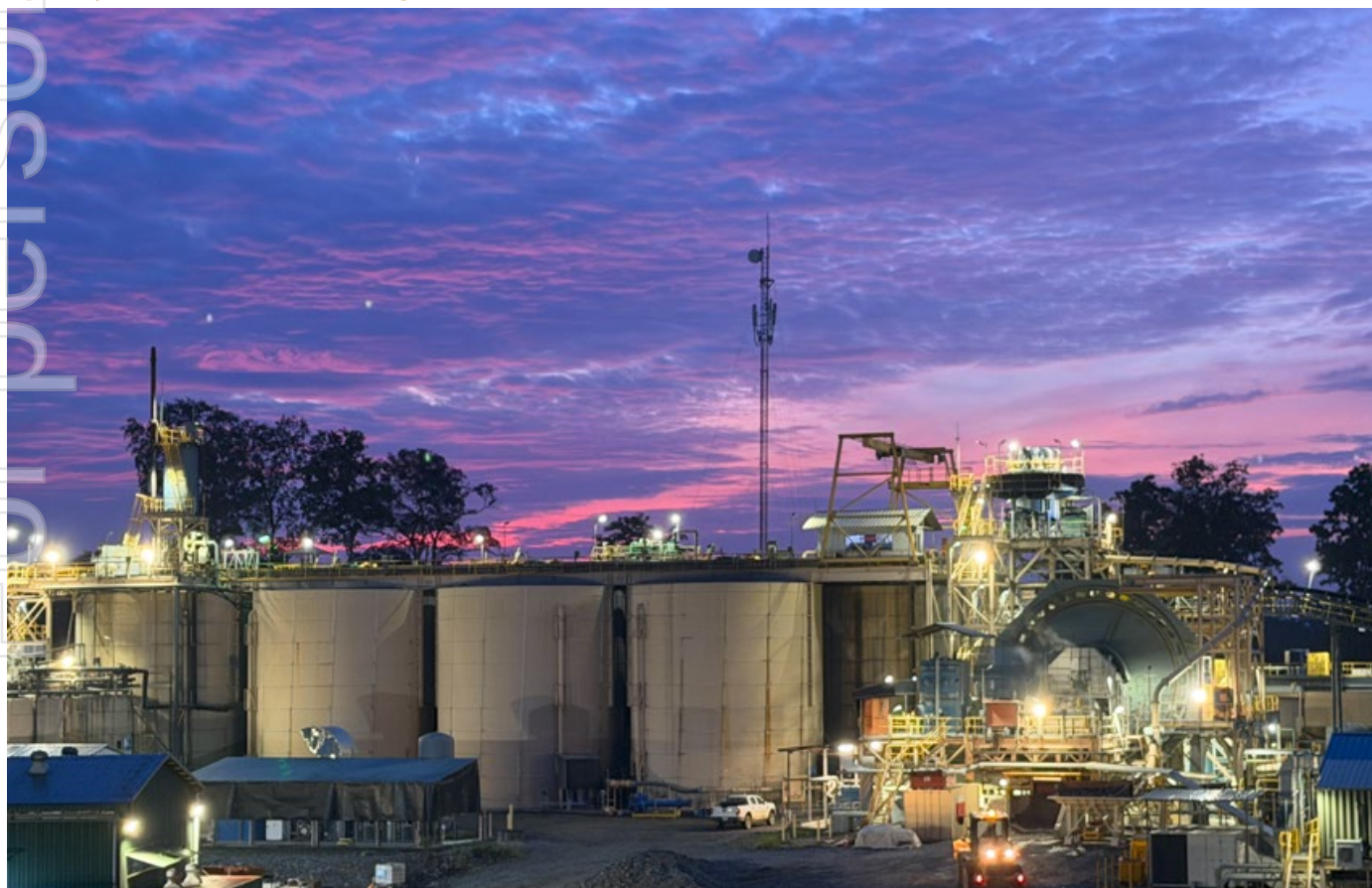
Figure 1 | Sunrise over Okvau Processing Plant
