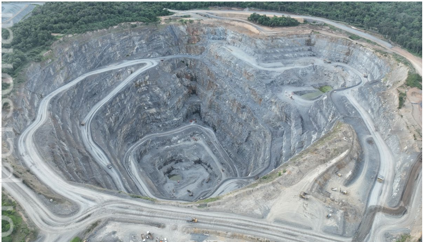
Figure 5 | Okvau Open Pit at July 2026
