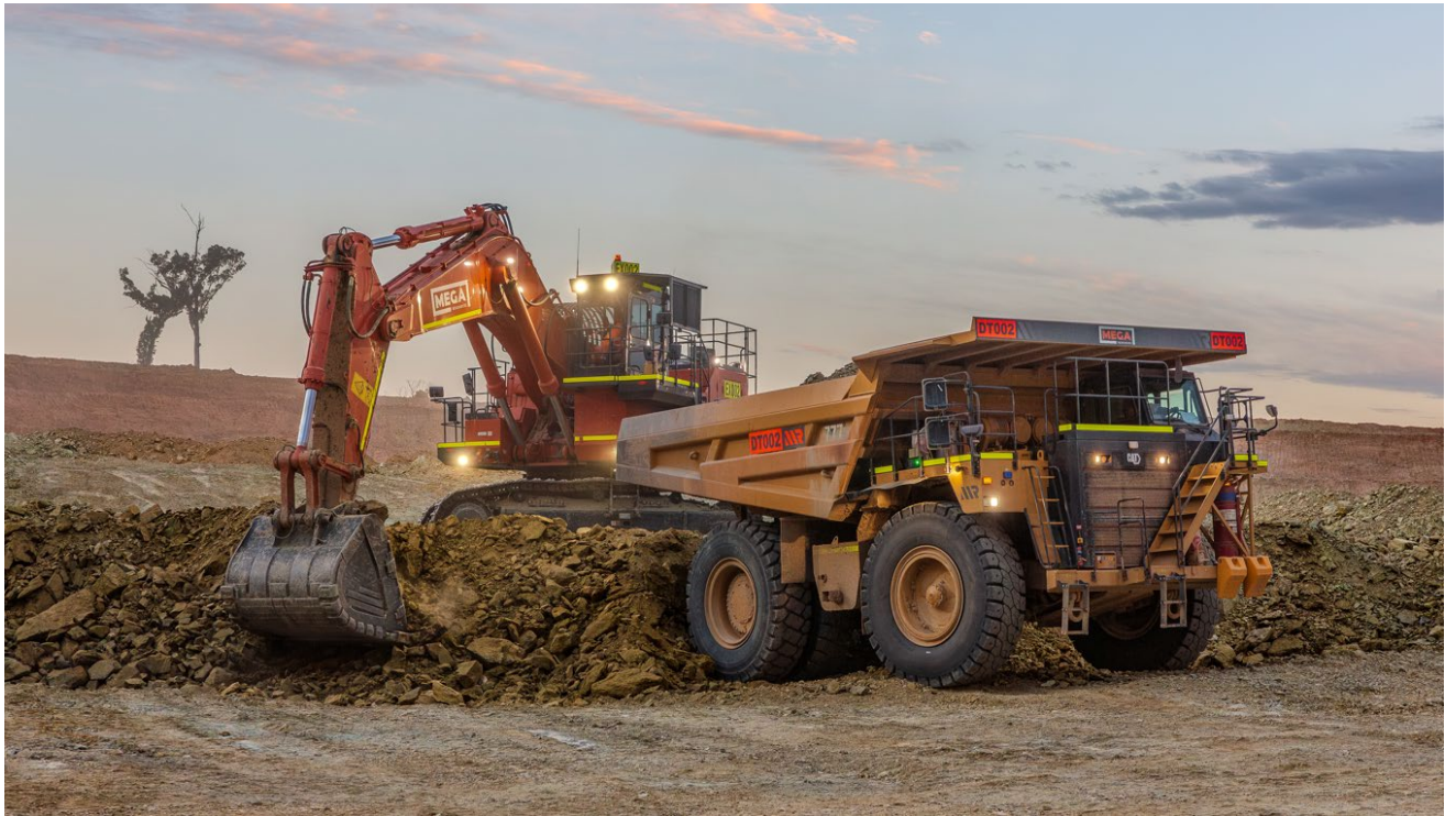
Image: MEGA Resources Excavator for use at Johnson Range
