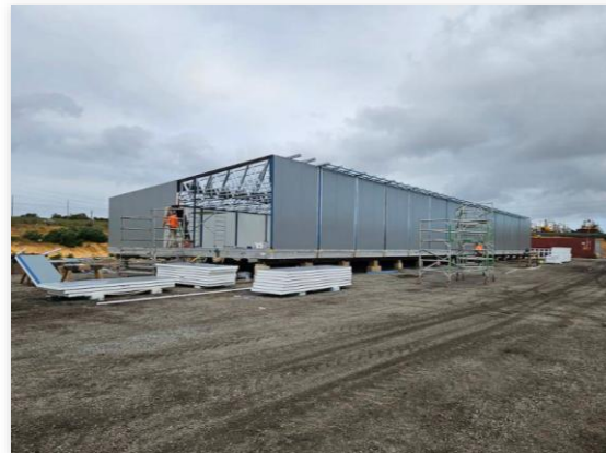
Permanent MSA 1 building construction
