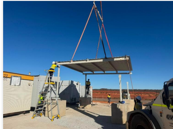
Project offices on-site works
