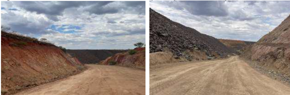
Figure 2 – Re-establishment of the Groundrush pit ramp to the decline portal location
