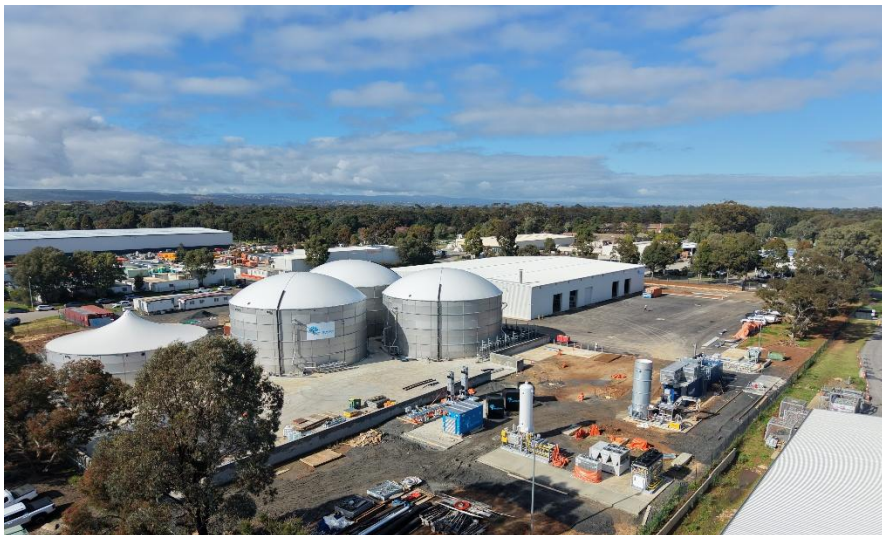
SA1 Salisbury Bioenergy construction
