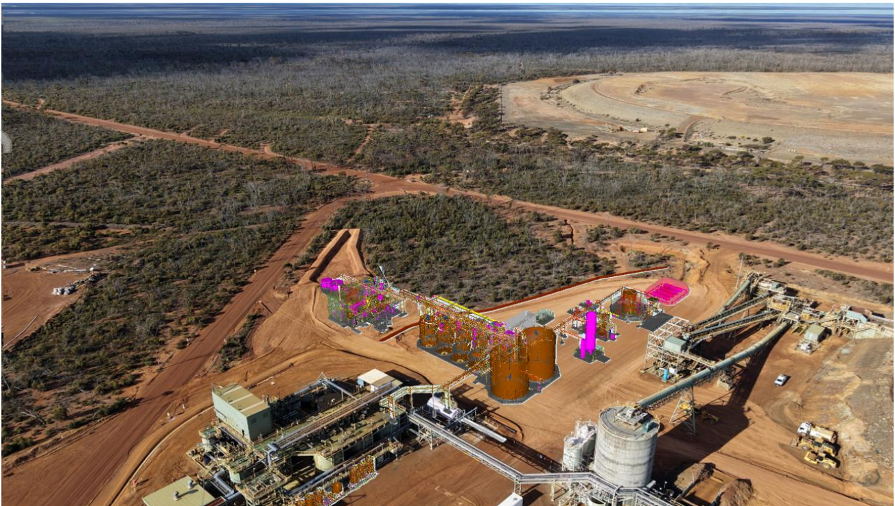
Figure 1: Existing CBC infrastructure with site earthworks completed for the new carbon in leach circuit (rendered)
