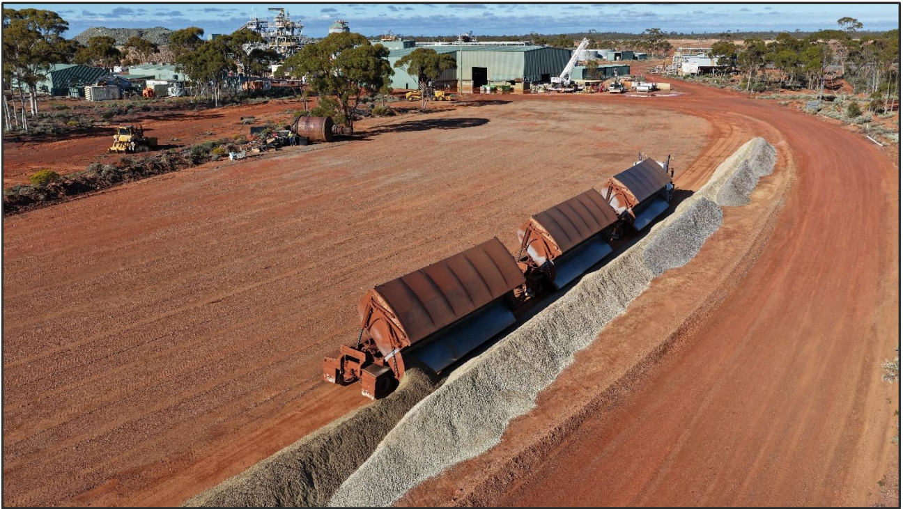
Figure 2 – CHS Mining Services commencement of select fill
