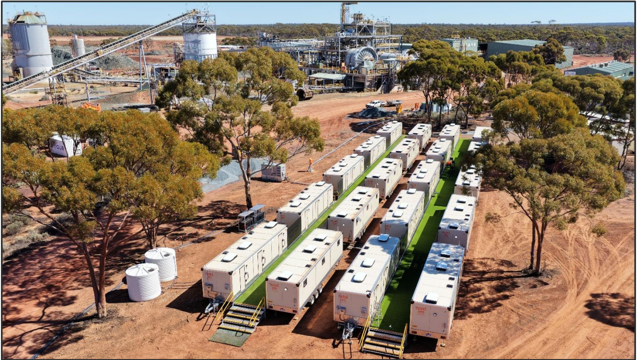
Figure 4 – BSHP Construction Camp Stage 2 – 57 Rooms
