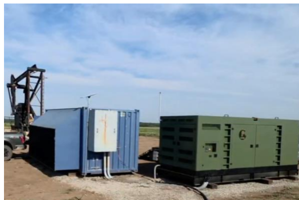
Figures 1 & 2: Initial Gas to Power installations at Charlie #1 Well
