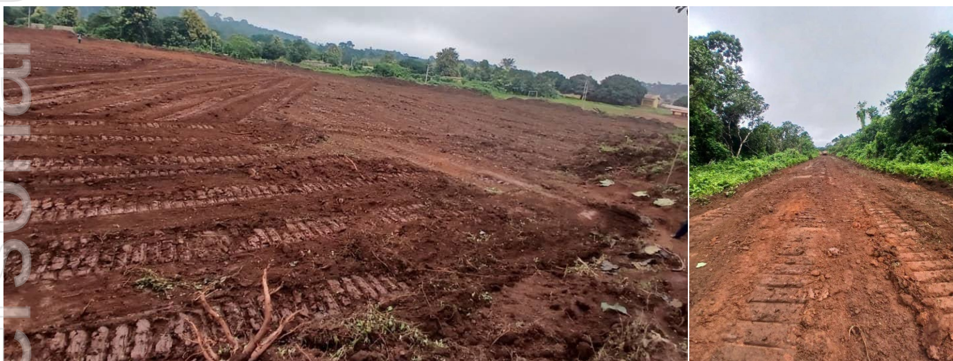
Figure 6 Bondoukou. Clearing designated parcel of land and road repairs for the Dingbi Village community within the Bondoukou Project area.
