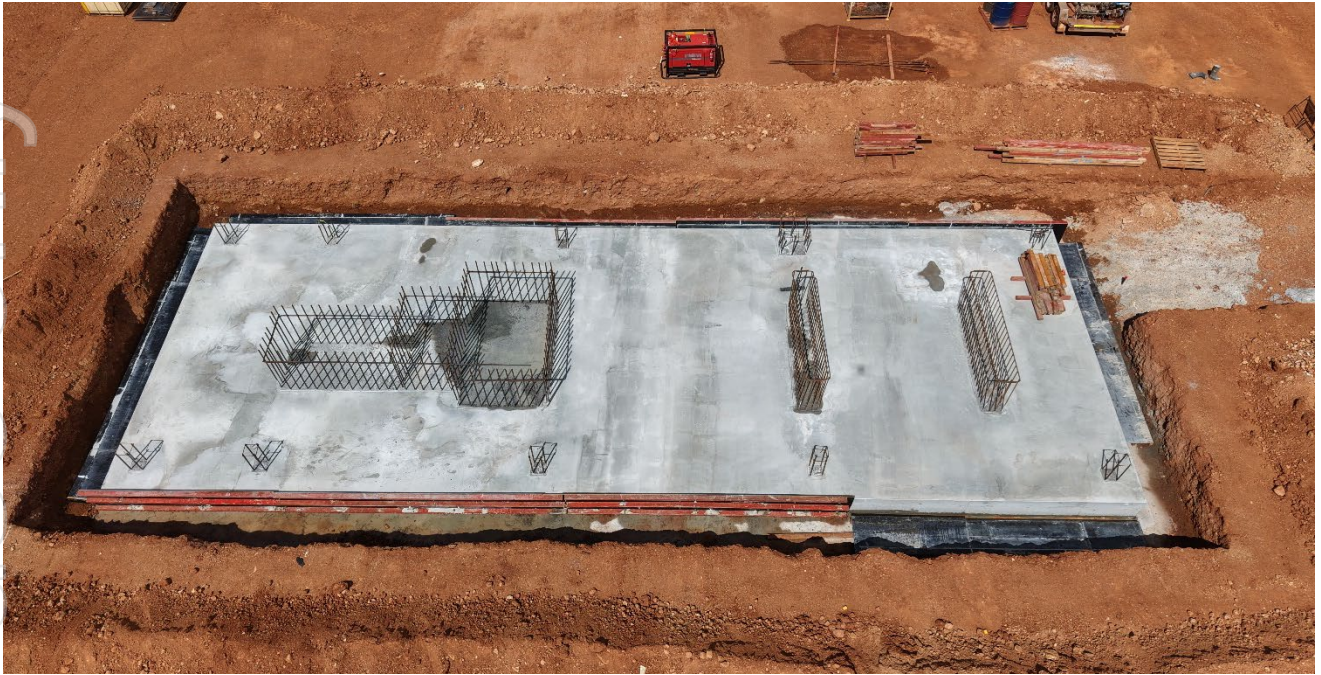
Figure 5 – ISAMill foundation poured
