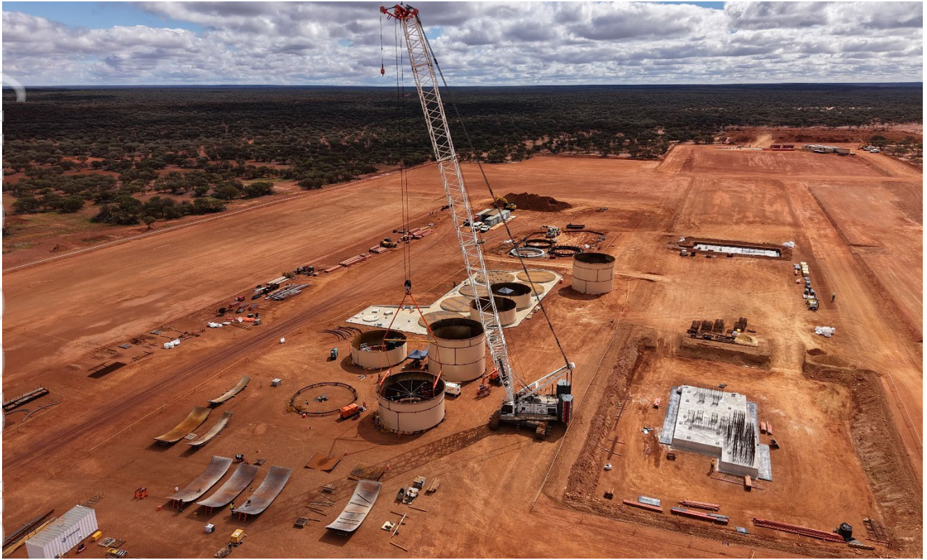
Figure 1 – Progress of construction on site – looking South
