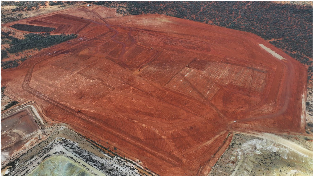
Figure 8 – Tailings Storage facility
