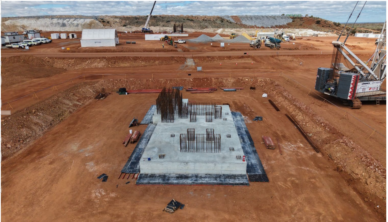
Figure 4 – Ball mill foundation poured
