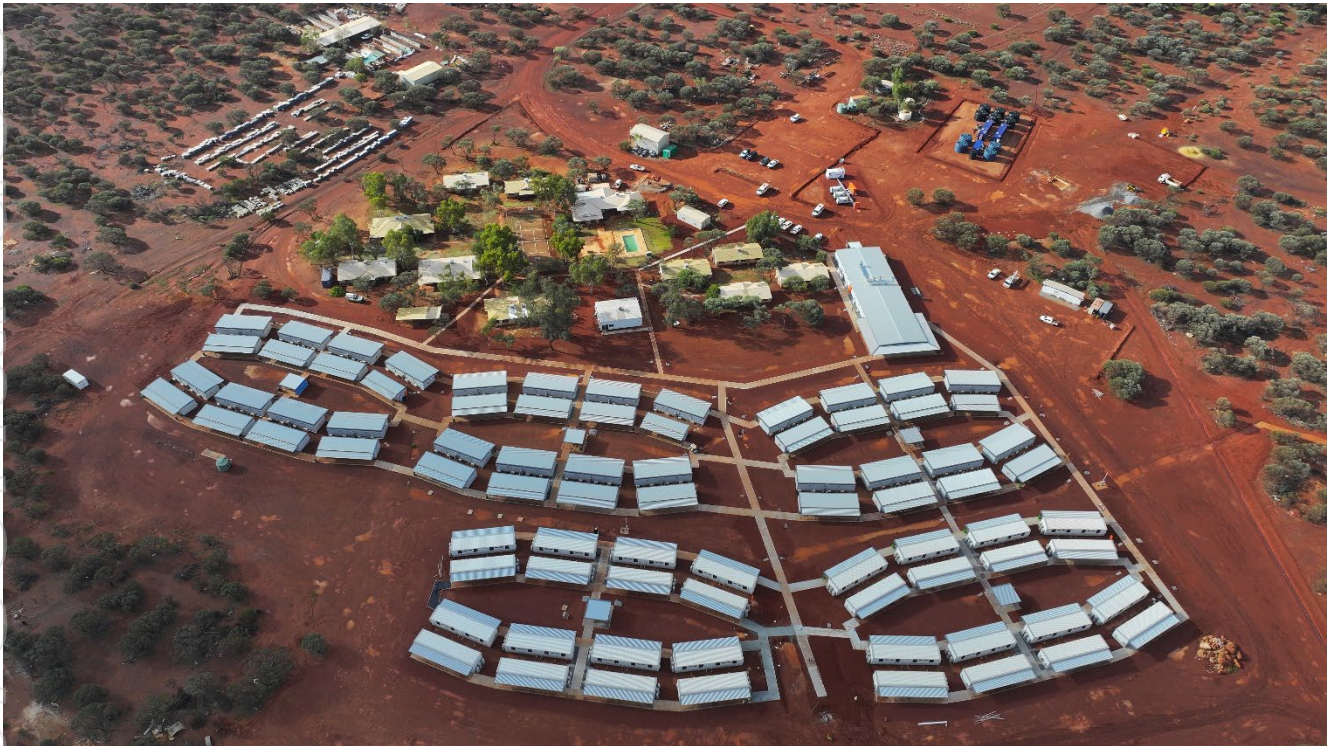
Figure 10 – Youanmi 351 room camp facility
