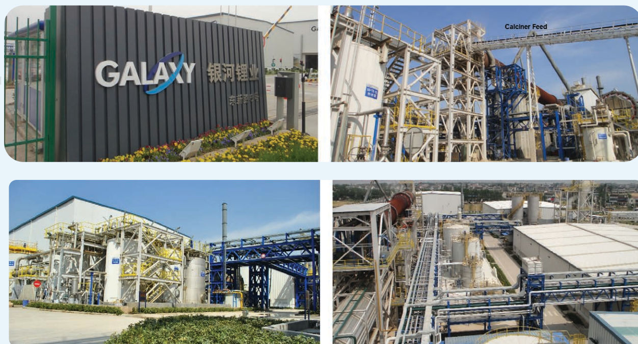
Figure 10: Galaxy Jiangsu Lithium Carbonate Plant
