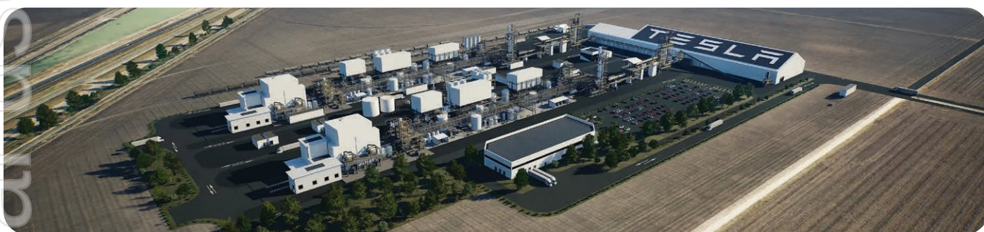
Photo: Tesla's Lithium refinery in Corpus Christi, Texas
