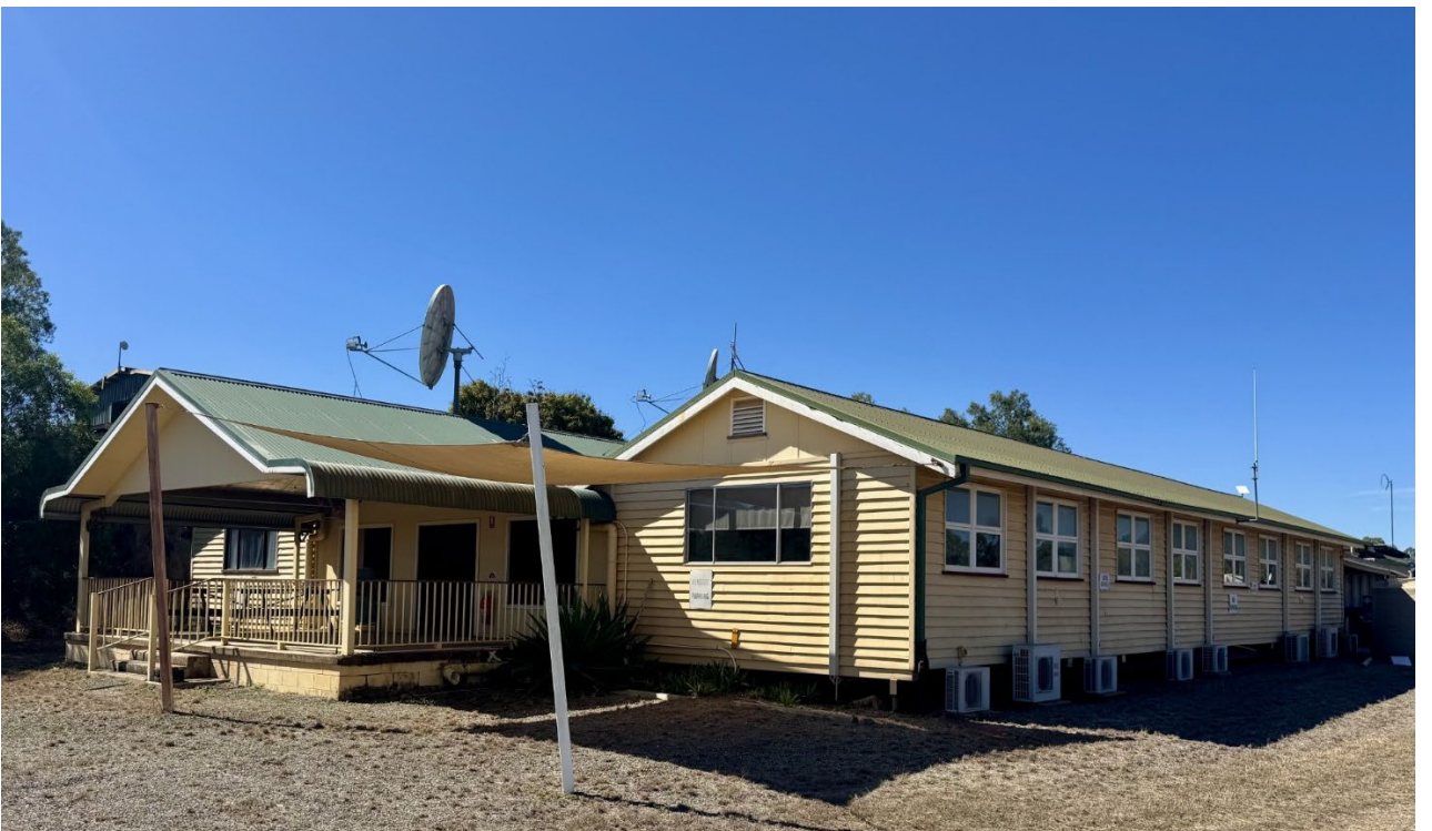
Figure 9: Recommissioning of site office complex.
