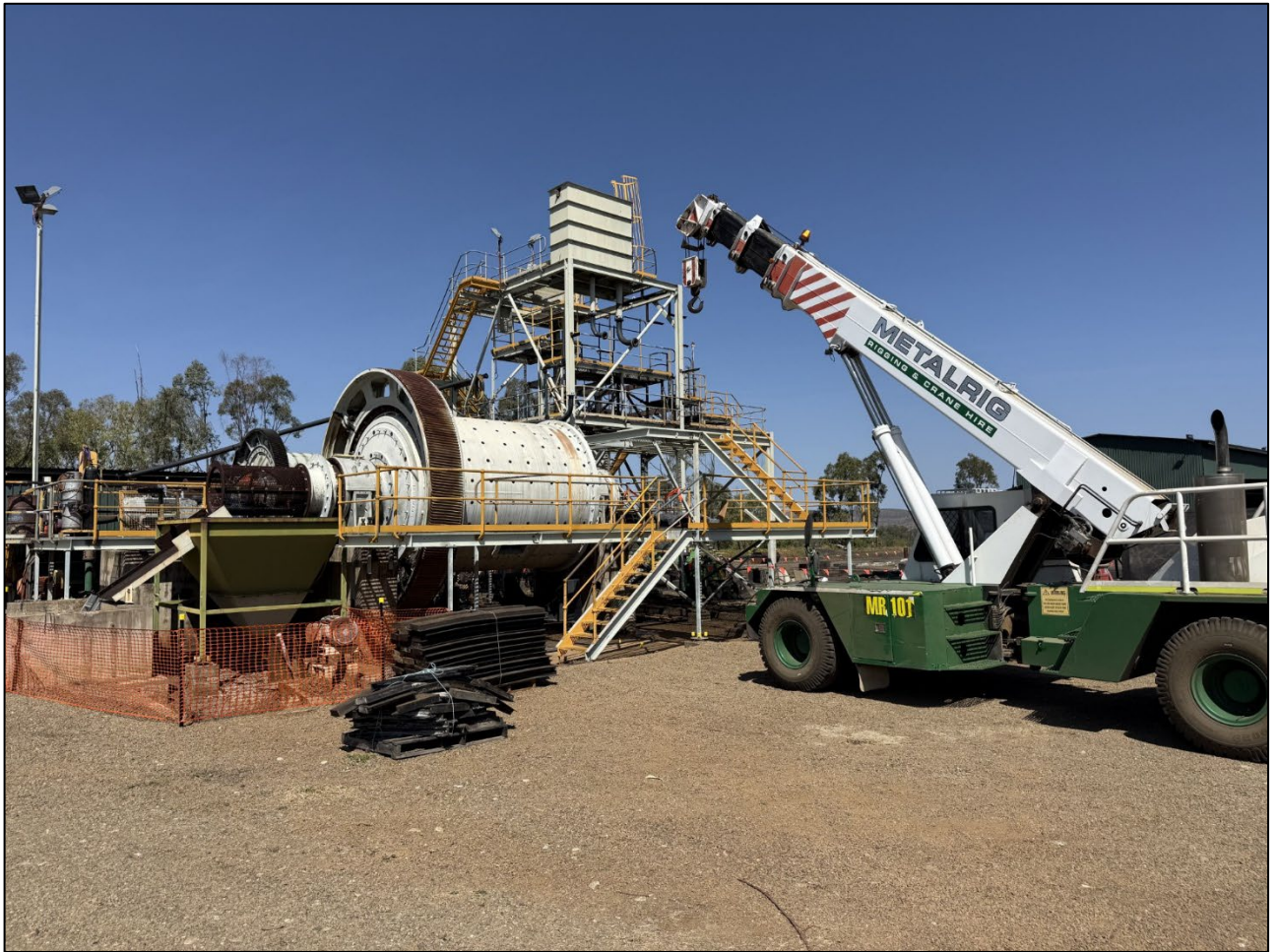
Figure 4: Liners removed from ball mills and being craned out on 13 August 2026.
