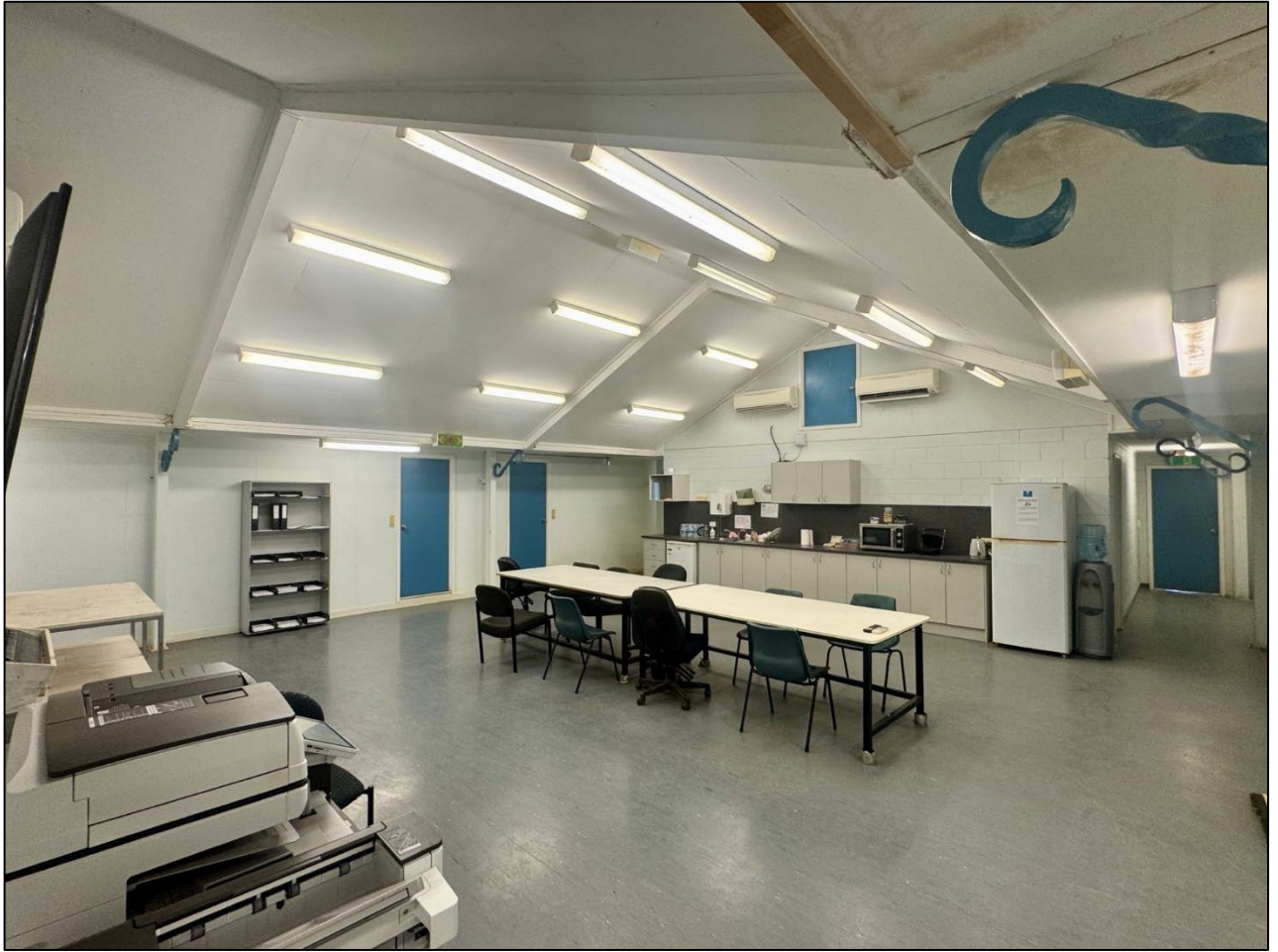
Figure 8: Recommissioning of site office complex.
