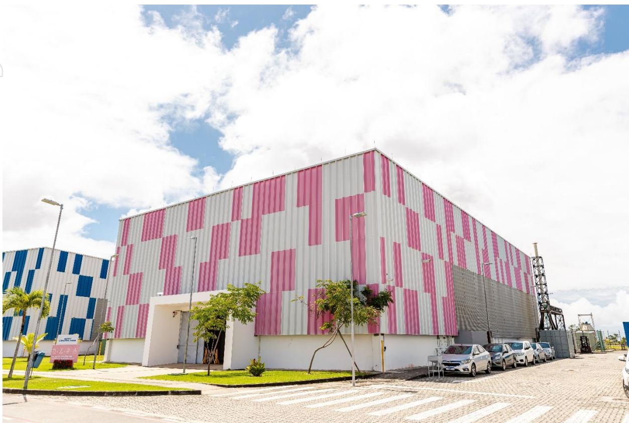
Figure 2: BRE Pilot Plant exterior.
