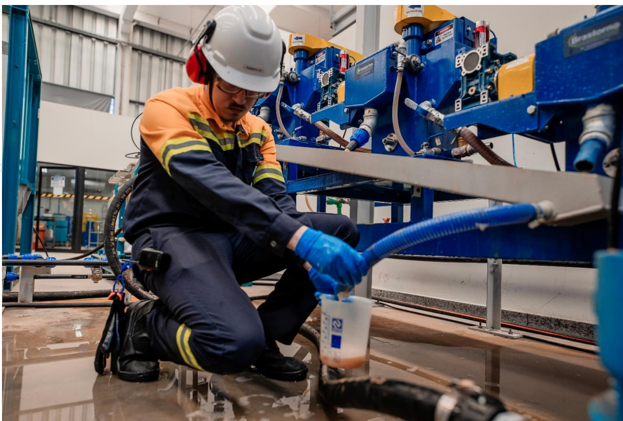
Figure 11: Process sample collection during commissioning.
