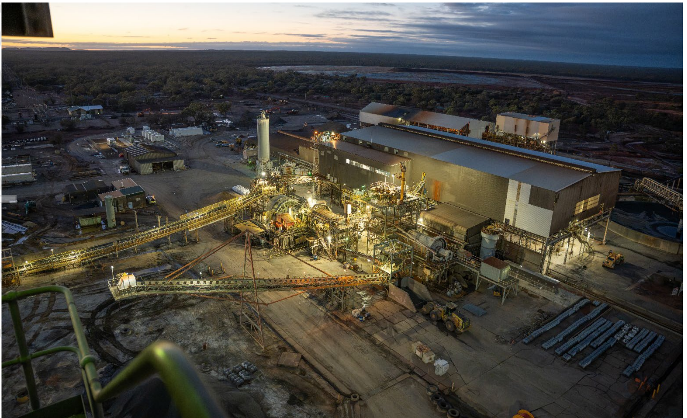
Figure 1. Endeavor combines a substantial underground mining system with existing shaft and decline access, an installed 1.2Mtpa processing plant, grid power, water, rail infrastructure and other established mining assets.
