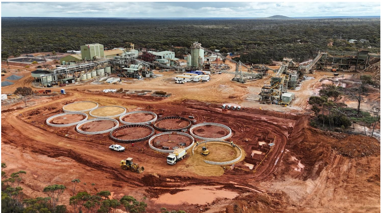
Image 3: CIL Tank construction - Lake Johnston Processing Facility
