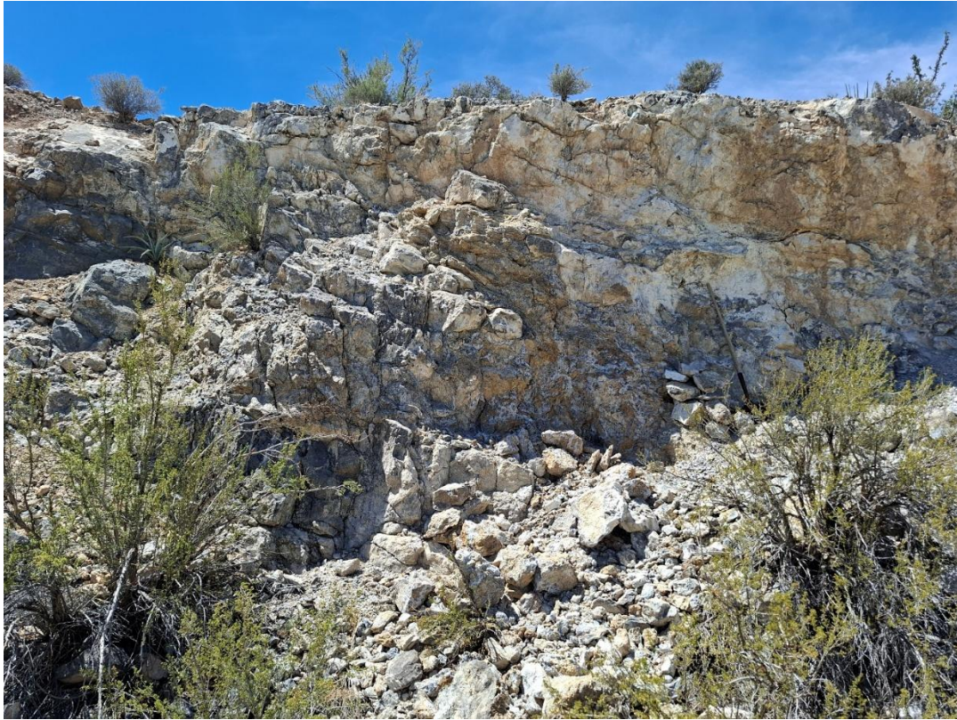
Figure 3: Fluorite Mineralisation in wall of West Pit
