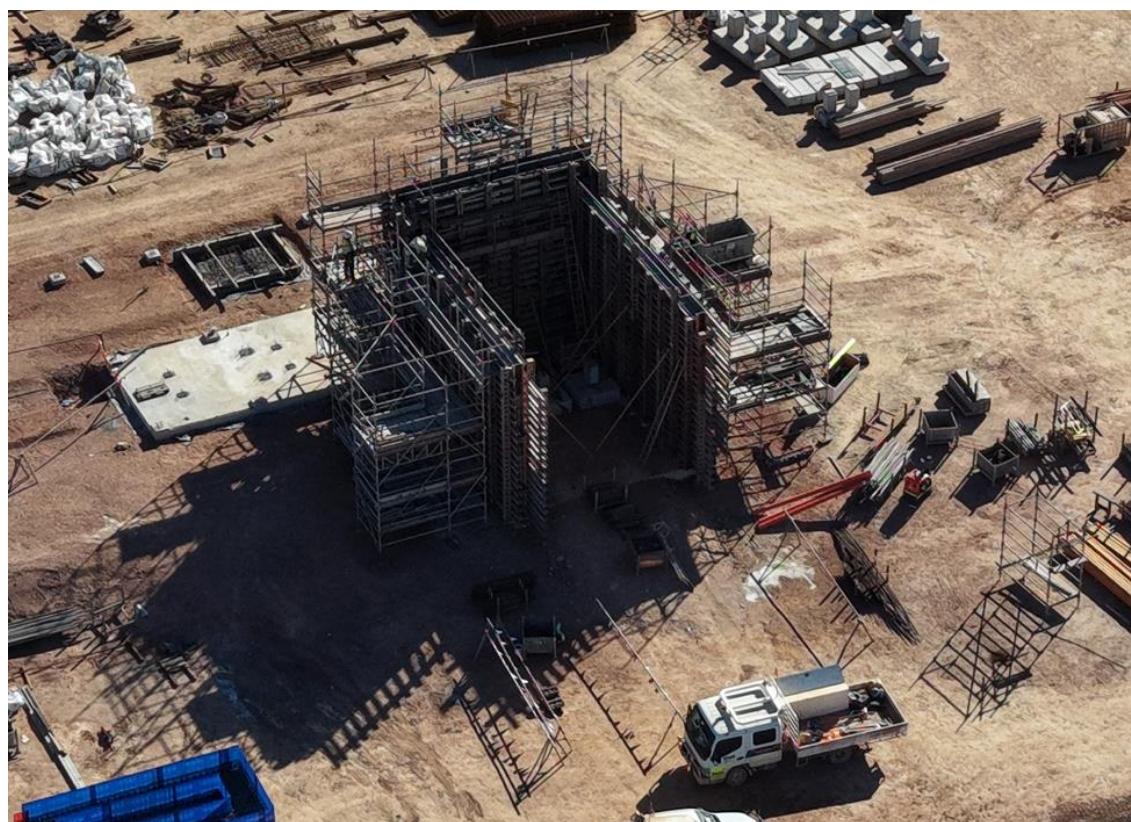
Figure 5: Surge bin and wall foundations
