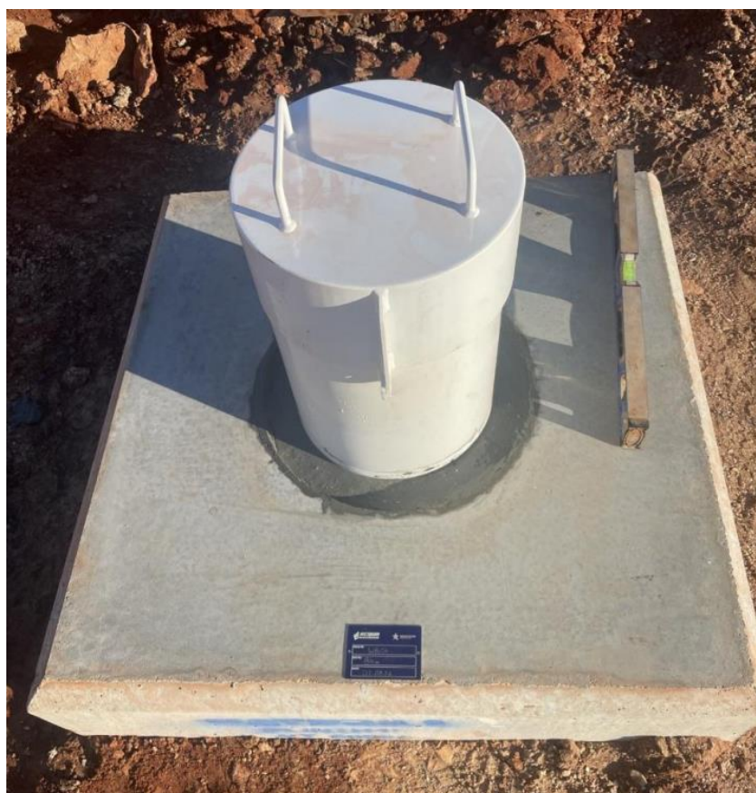
Figure 7: Completed bore – ready for pipework system installation
