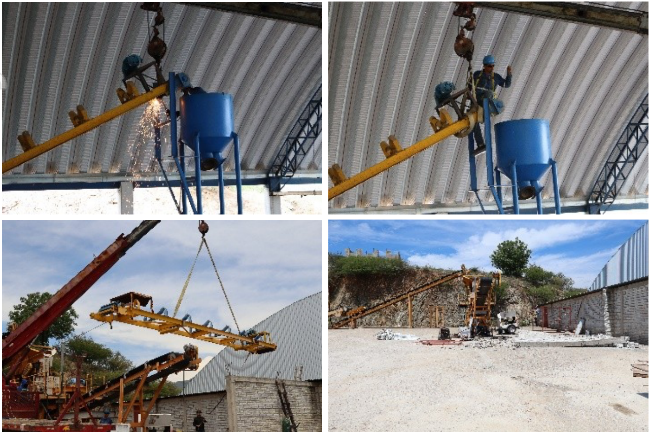
Figure 4: Removal of legacy barite conveyors and dust collectors, and clearing of the crushed-ore stockpile area
