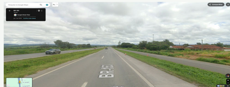
Condition of State Highway BR-153 (Belém-Brasília Highway), the main connection corridor to Goiânia.
