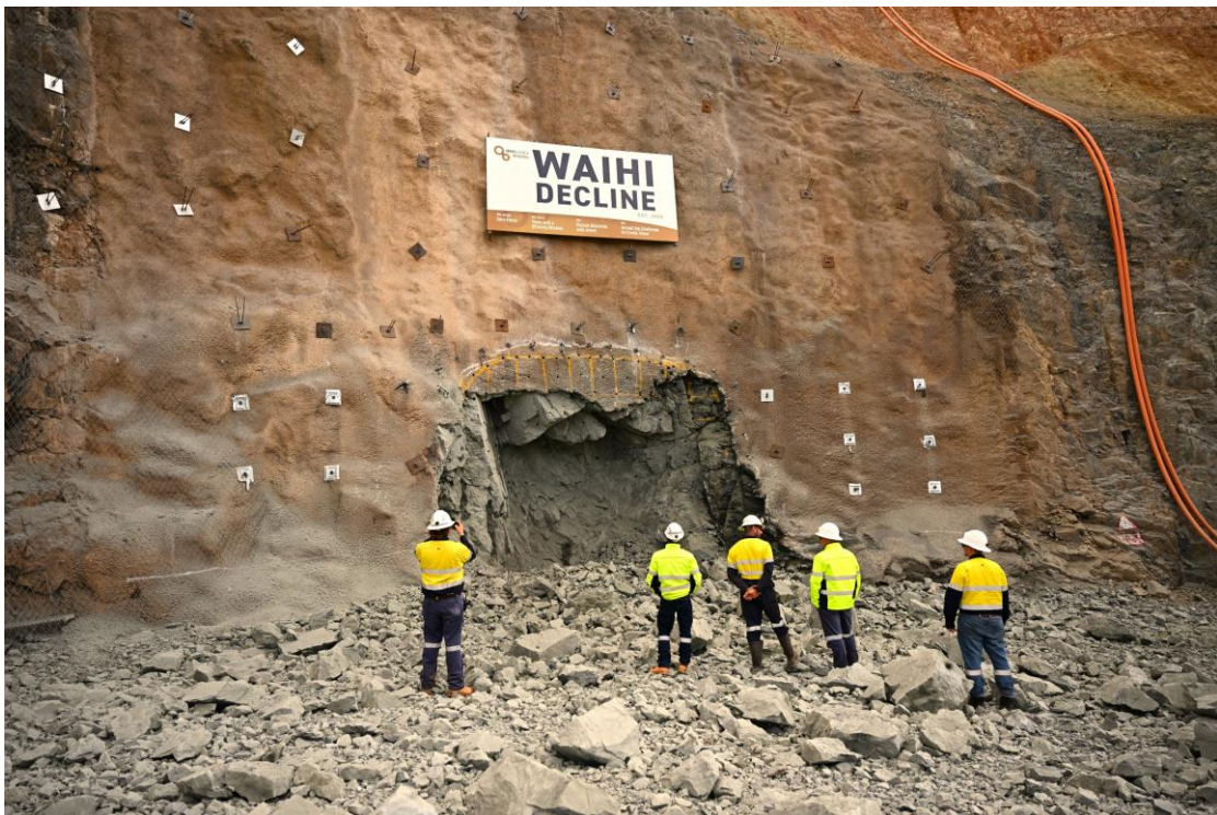
Figure 3 - Inspection of the first cut, Waihi Portal
