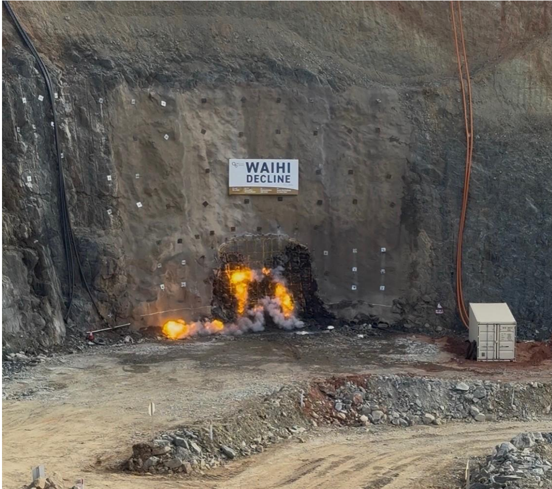
Figure 2 - First Firing, Waihi Decline
