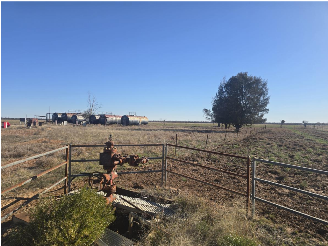
Figure 4 Looking from Riverslea-3 to the tank farm
