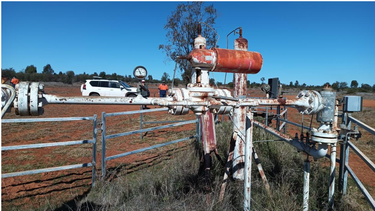
Figure 6 Managing Director scoping out wellhead works ahead of tie into Silver Springs with wellhead pressure reading of 1,000 psi
