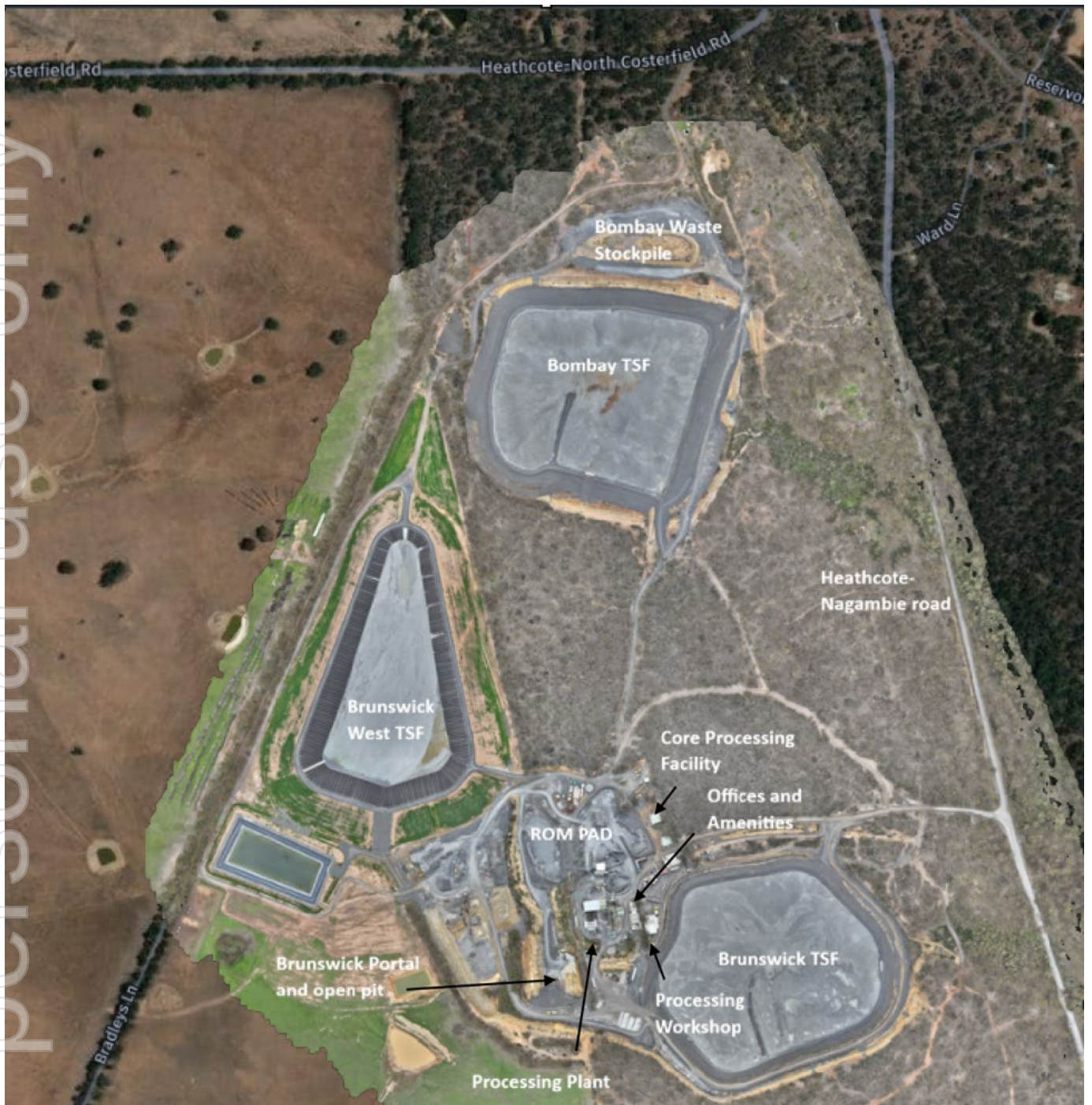
Figure 14: Brunswick Site, including processing plant, offices, exploration facilities, and tailing storage facilities
