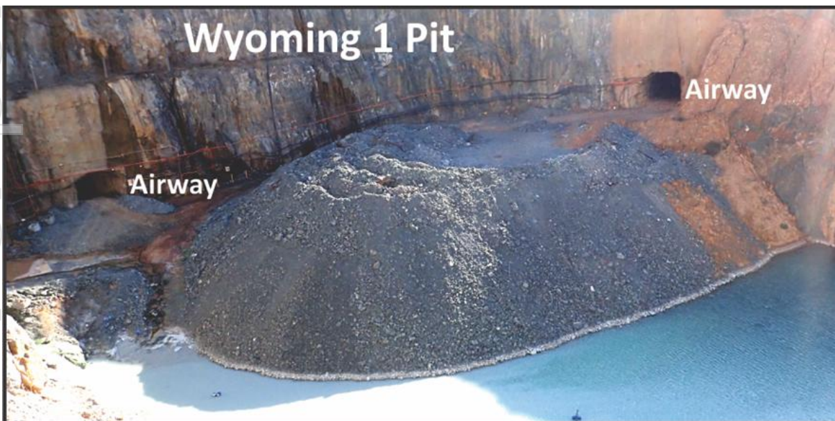
Figure 16-6: Additional airways in the Wyoming Pit
