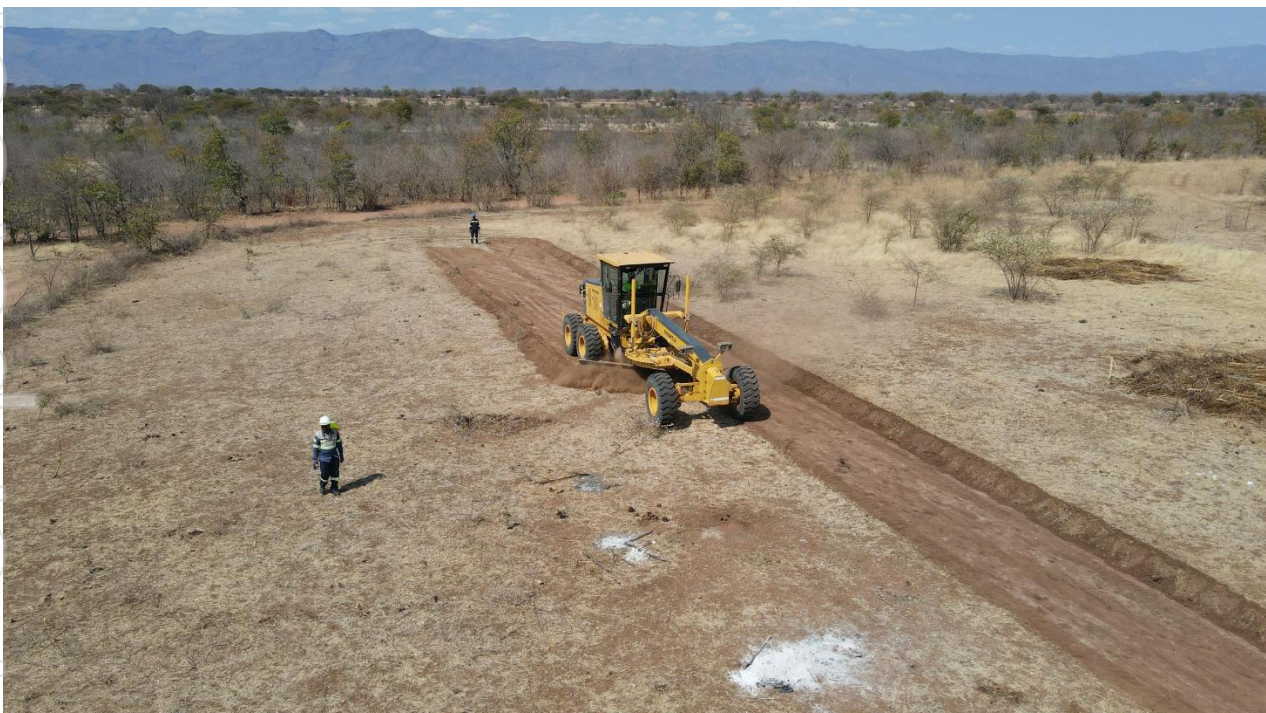
Figure 4 - Musuma-1 Wellpad ground breaking
