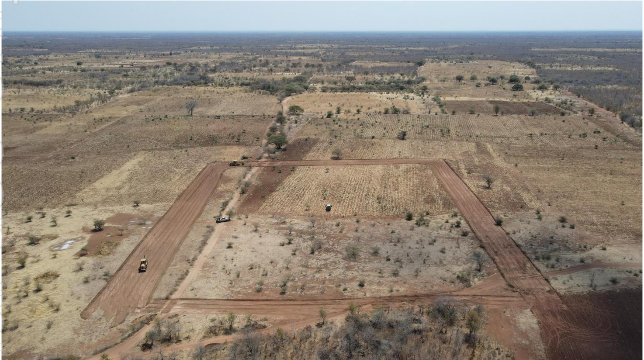
Figure 3 - Musuma-1 wellpad preparation
