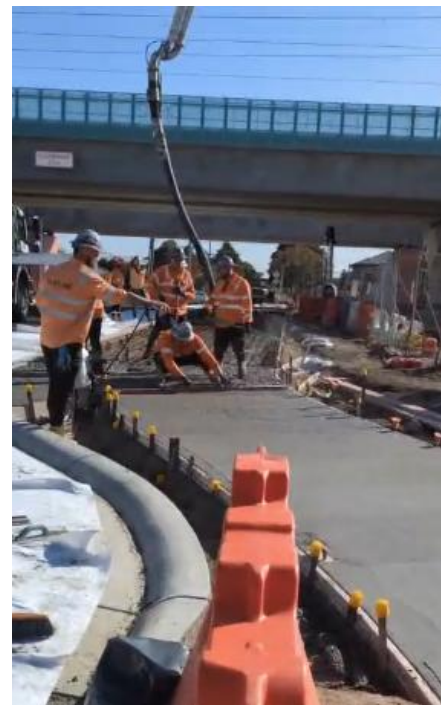
Figure 1: Concrete containing G360's MKX being placed by Eifers as part of footpath pavement works in Newport, Melbourne.
