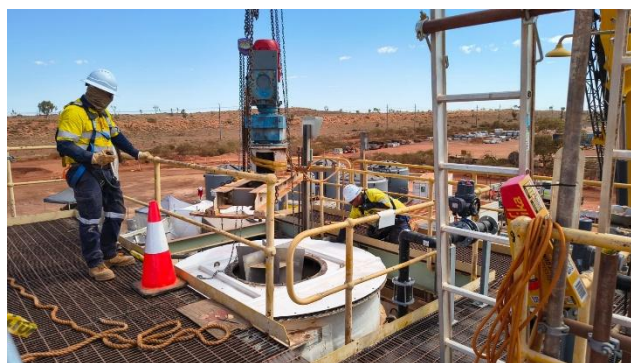
Mixer blade and rotor lifted and installed
