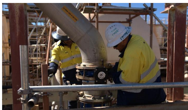
Detailed pipe installation
