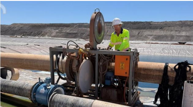
Welding main pipeworks
