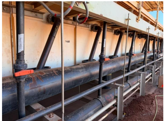
EW pipework installed
