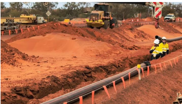
Process water lines being buried
