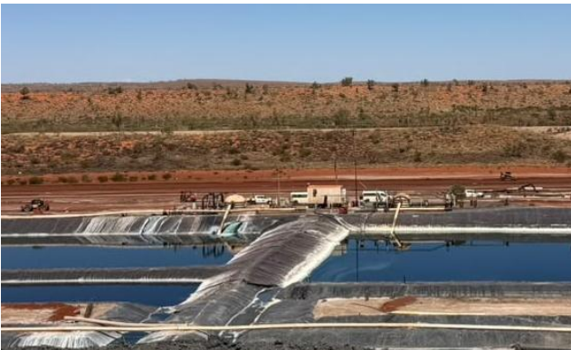
ILS2 and PLS2 pump station commissioning
