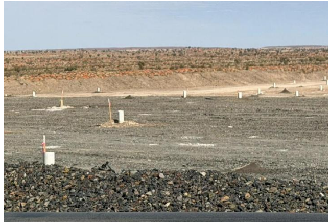
Future production areas drilled and cased
