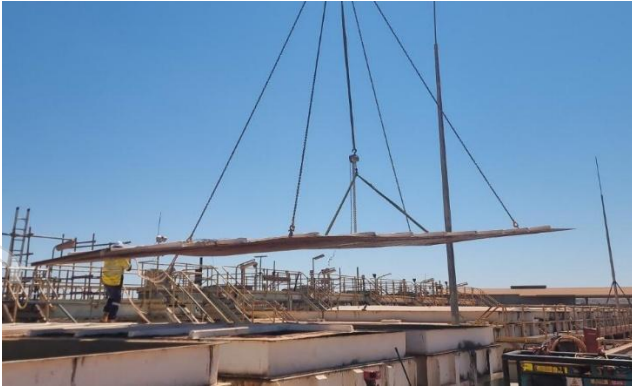
Settler tank lids lifted into place
