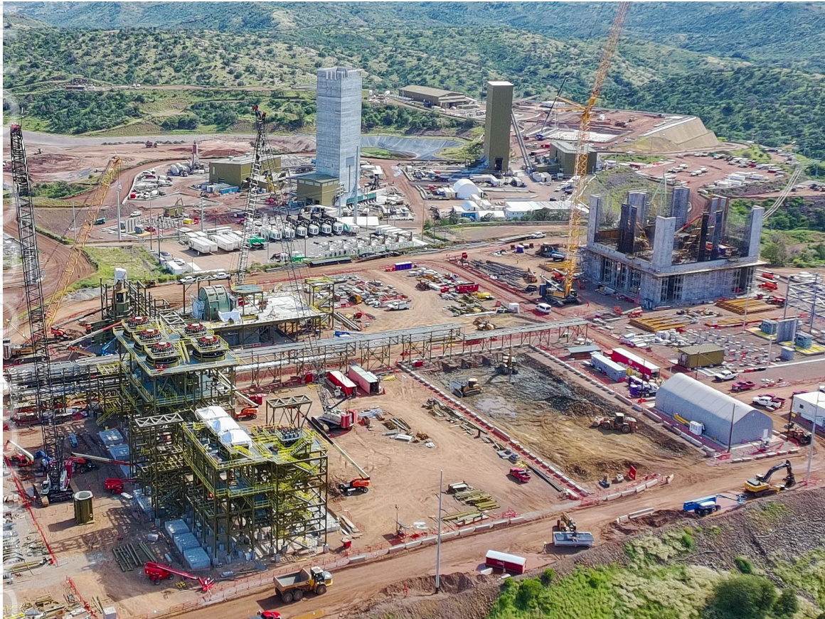
Taylor process plant construction (looking north)
