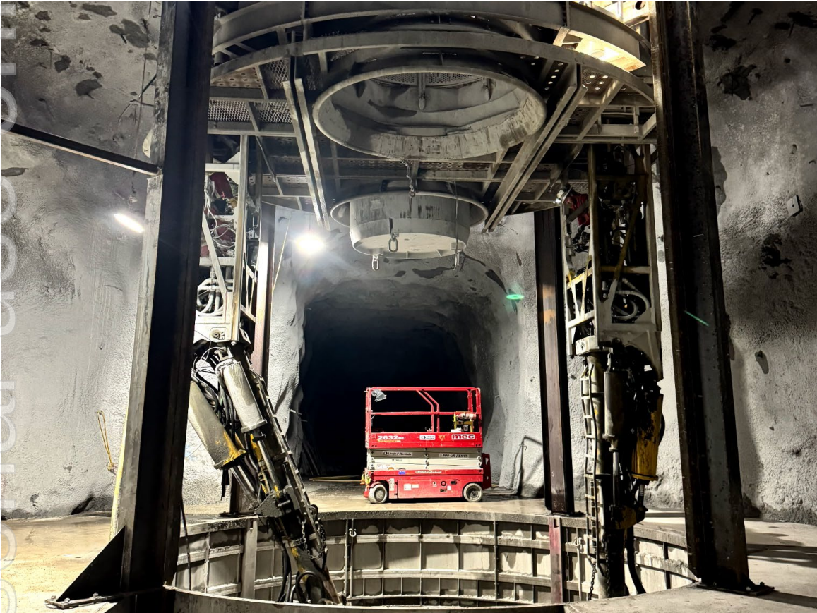
Main shaft development
