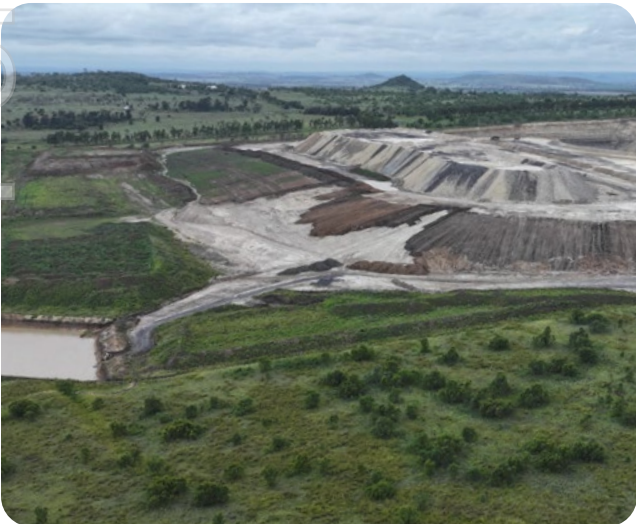
Rehabilitation at Willeroo Pit, New Acland, January 2026.
