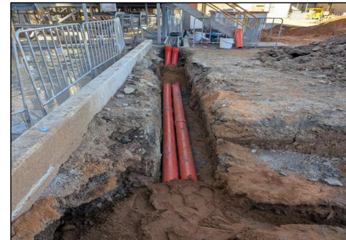
August 2026 – electrical tie-in
