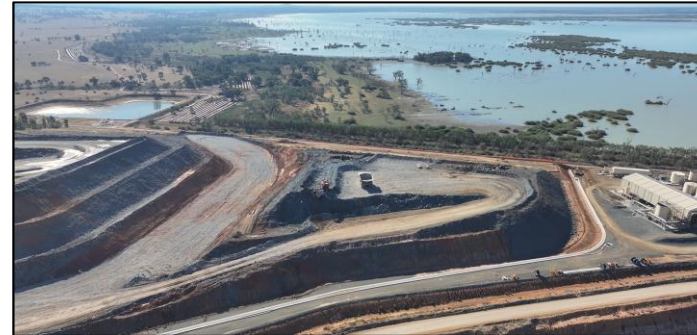
May 2025 – Pre-North Lake Protection Bund
